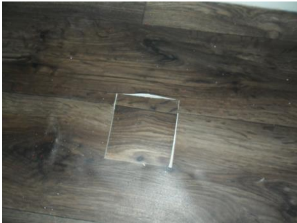
Patch to vinyl Floor
